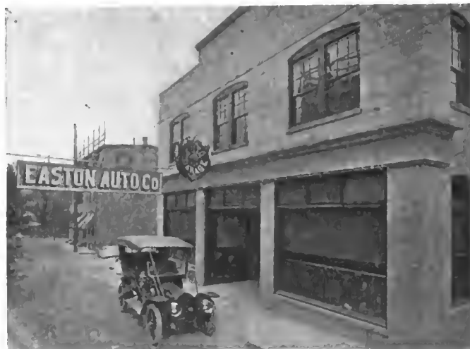
New Fireproof Garage of Easton Auto Co., Easton, Pa.
